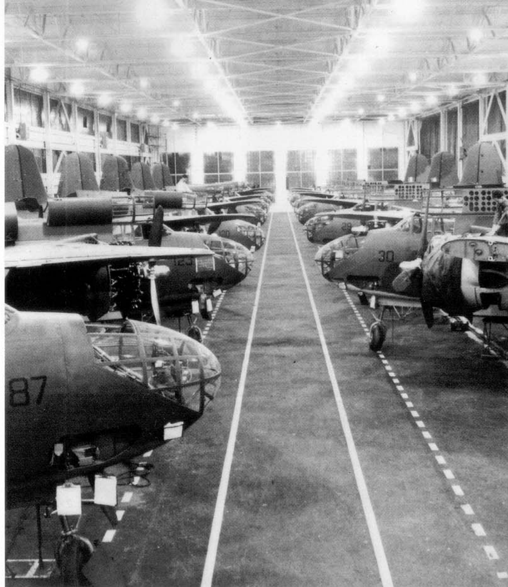
The largest portion of A-20 production took place at the Douglas Santa Monica plant where 808 were produced. Boeing built an additional 140 at their Seattle plant under license from Douglas. There were only minor differences between the two types, mainly in the electrical system and the exhaust and intake arrangement. (USAF)
